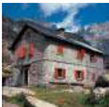
Prudenzini mountain hut in Val Savio
