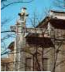
Facade in via Gramsci designed by Egidio Dabbeni
